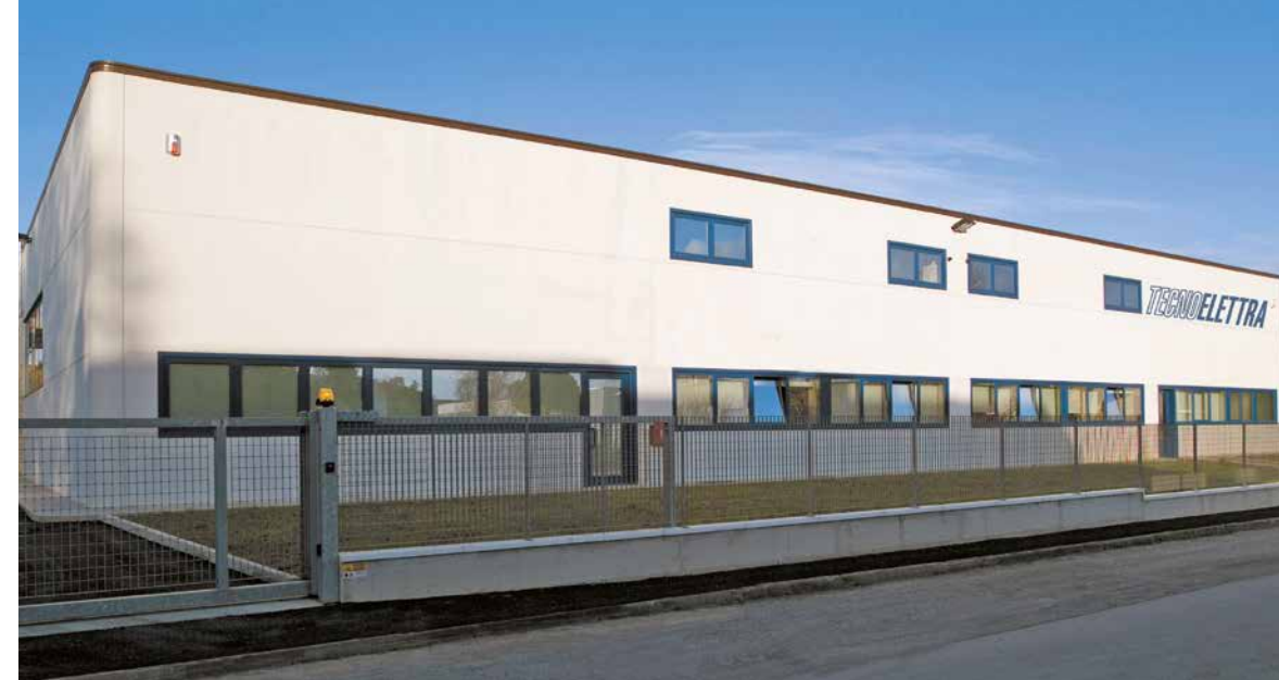
Tecno Elettra headquarters in Monsano, Italy.
